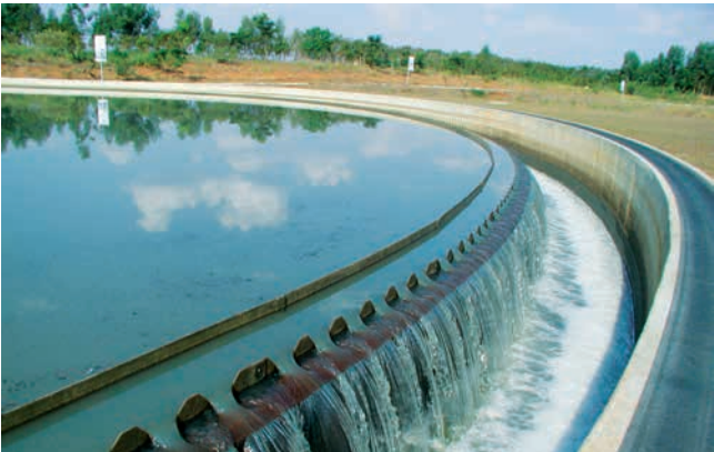
Municipal wastewater treatment
