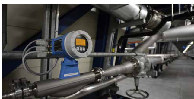
Coriolis-based density measurement in the sludge conditioning process with a Promass device
