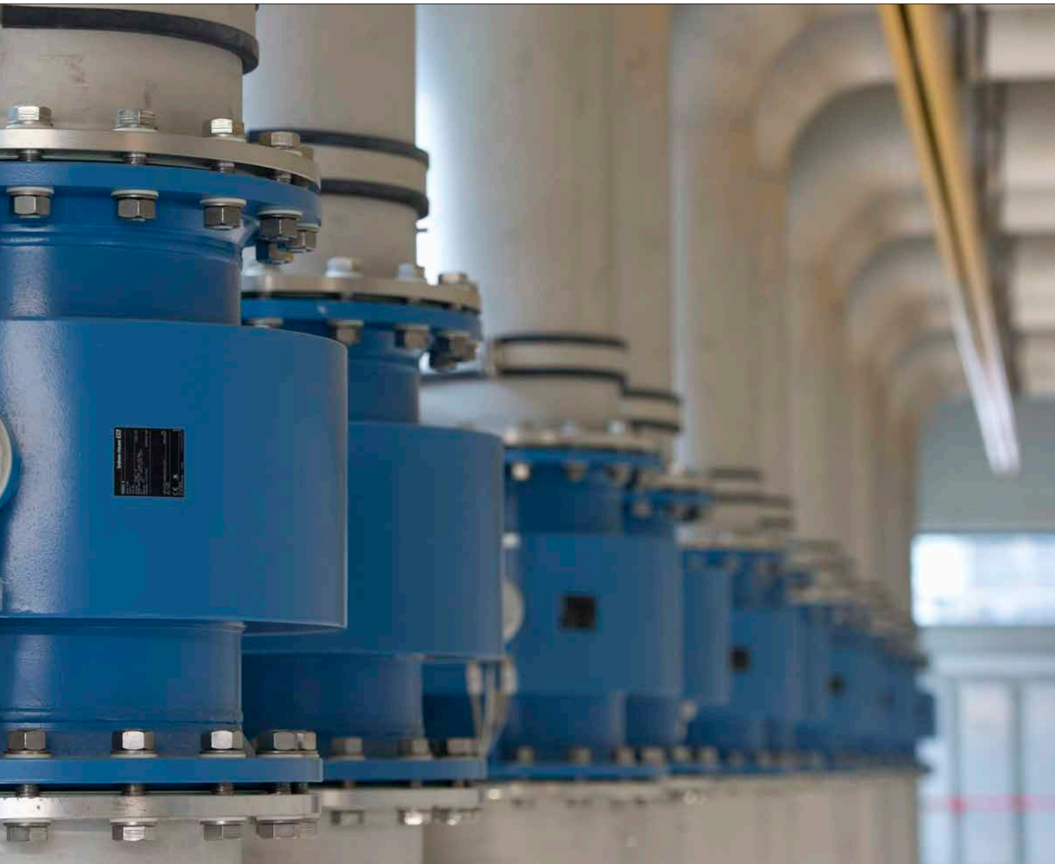
Flow measurement of water, wastewater or sludge: The electromagnetic induction method of flow measurement is the standard
